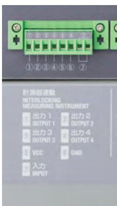
Instrumentation interlock terminals
